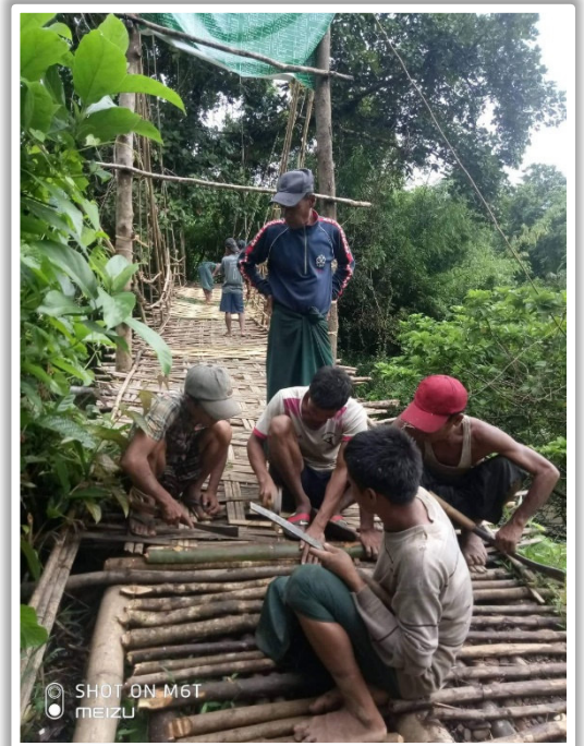
Brückenreparatur in Pyin Taung (Rakhine)
